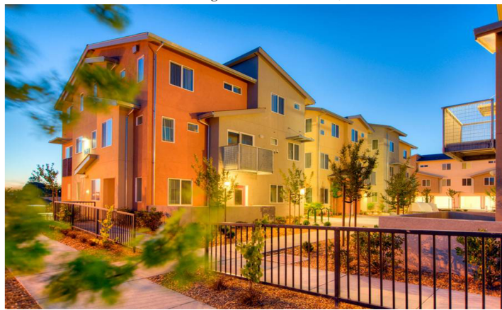
Two-and-three-story apartments and townhomes rise above ground floor studios and fully accessible units at Amorosa Village.
